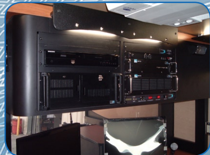
VIEWING ROOM WITH ELECTRONIC COMPONENTS MOUNTED ABOVE THE DESKTOP & ADDITIONAL COUNTERSPACE
