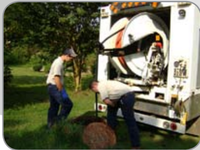
PERFORM PIPE CLEANING
